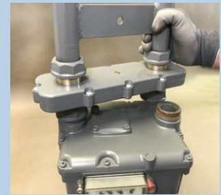
4 Connect the inlet side of the new meter & install a nut plug in the outlet.
